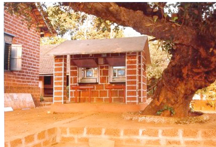
Figure 2: Photo of an MIE kiosk, Sindhudurg
